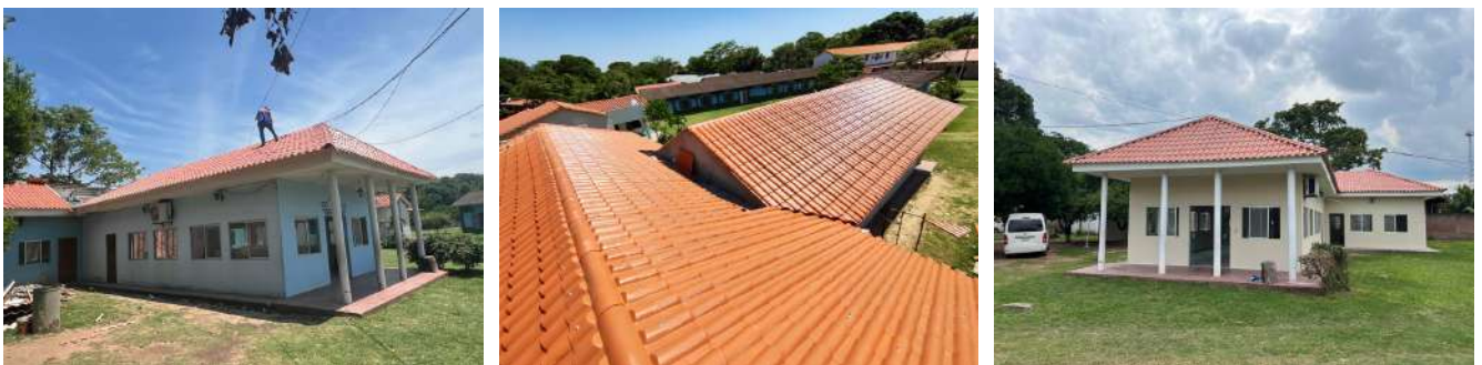
During and after shots of the maintenance and upgrades one on the chapel.
