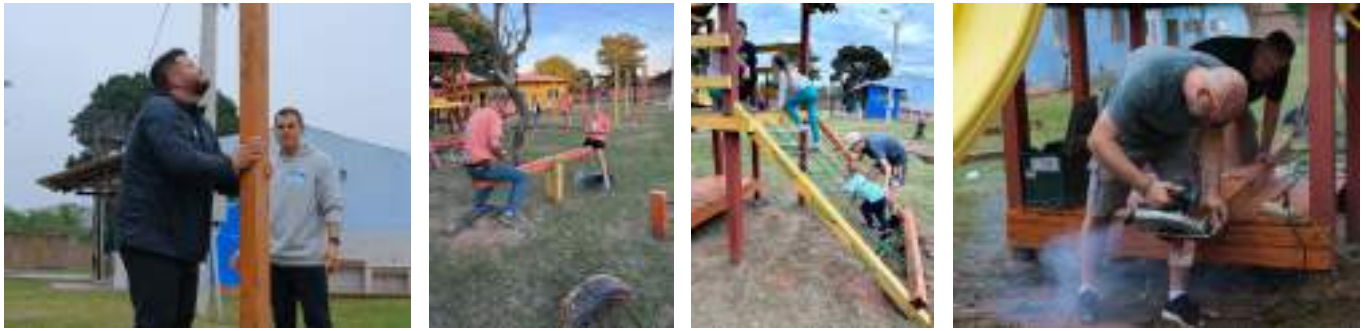
Far left: Drake and Matt help remove the damaged swing set in a spontaneous project to repair the playground area. Center left: Dave and Melanie test out the repaired see-saw. Center right: The repaired climbing net. Far right: Dave and Christ work on replacing broken and rotted boards.
